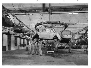
large amounts of interchangeable parts were created and then assembled. This allowed massive improvements in efficiency and dramatic cost reductions.
